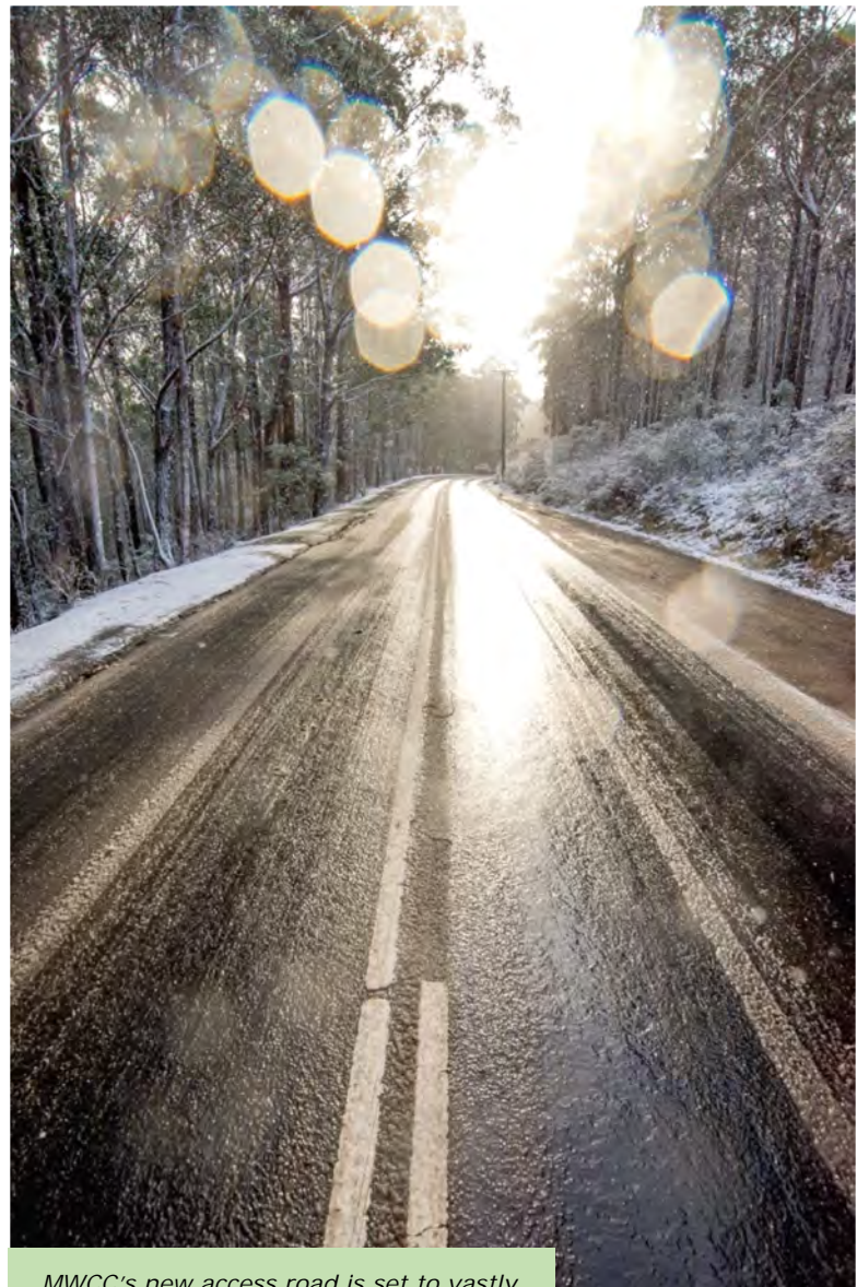
MWCC's new access road is set to vastly improve access for emergency services and utility organisations into the Park.
